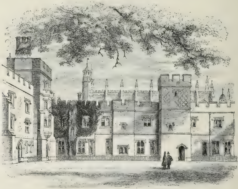
Fig. 34. North side of the range containing "Long Chamber," from Weston's Yard; from Lyte's "Eton College."
